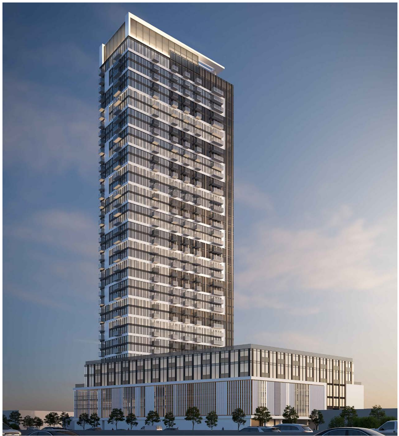
Looking east to 1515 Pickering Parkway, designed by Arcadis for Sevoy Developments
